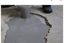
Pourable Polymer Modified Traffic Bearing Repair Mortar- TRM™ 200
