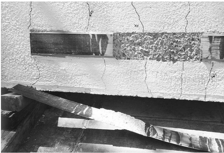
5.4 Close-up showing splitting within the prefabricated strip.
