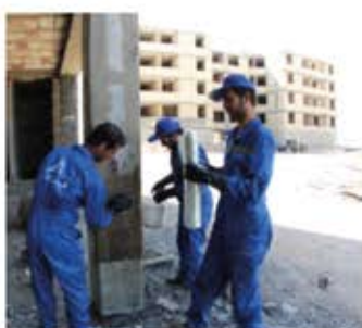
Glass wrap in plain, unidirectional and twill weave
