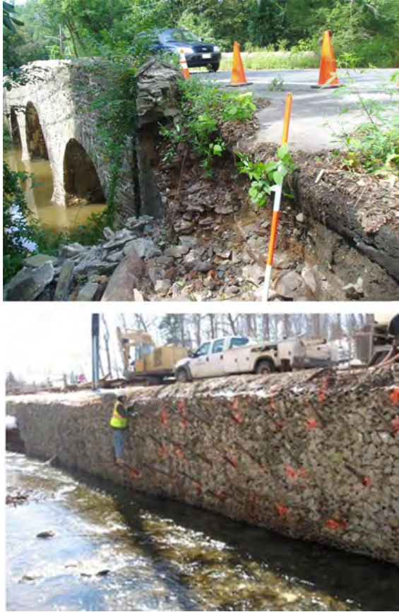
Figure 15.5 Rehabilitation of historic rock retaining walls with soil nails. Courtesy of GeoStabilization International.
