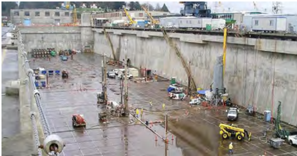
Figure 12.15 Re-leveling of the distressed floor slab of Puget Sound Naval Shipyard dry dock. Courtesy of Layne Christensen.
