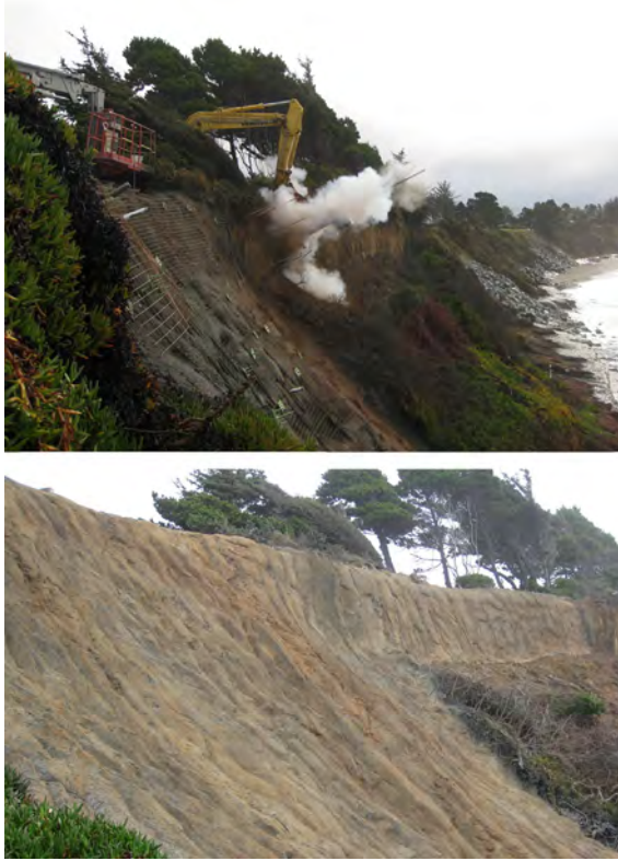
Figure 15.7 Stabilization of coastal bluff with fiberglass launched soil nails: Before and after stained shotcrete finish. Courtesy of GeoStabilization International.
