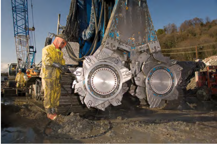
Figure 11.14 Cutter soil mixing apparatus. Courtesy of Malcolm Drilling Company, Inc.
