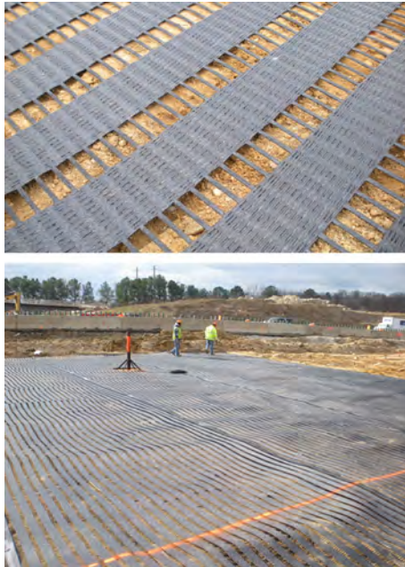
Figure 14.20 Application of high strength polyester/polyethylene geogrid for a new highway interchange. Courtesy of Maccaferri-USA.
