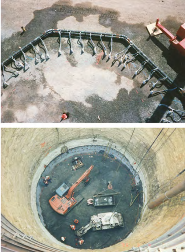
Figure 13.10 60 m (200 ft) deep, 18 m (60 ft) diameter shaft enabled by 90 m (300 ft) deep freezing, San Diego. Courtesy of Layne Christensen.
