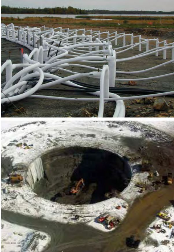
Figure 13.13 Shaft excavation in sensitive clay at Verglas mining project, Quebec, Canada. Courtesy of Layne Christensen.
