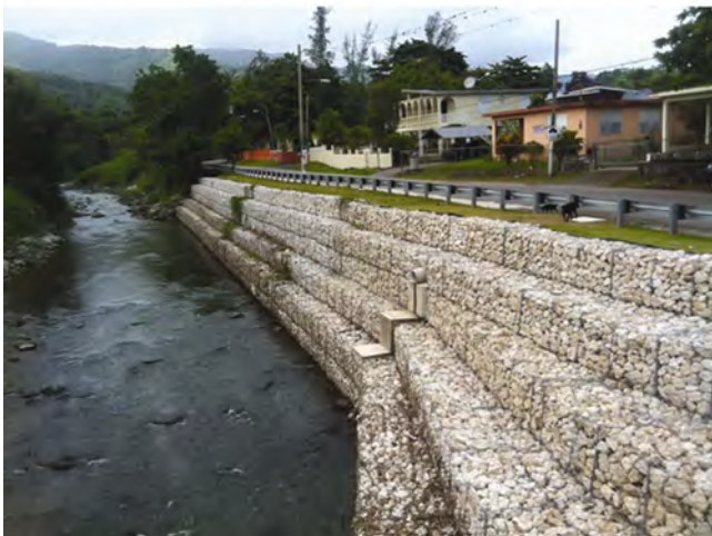
Figure 16.9 Gabion buttress walls for channel bank stabilization/protection. Top: Courtesy of Hayward Baker; Bottom: Courtesy of Maccaferri, Inc.
