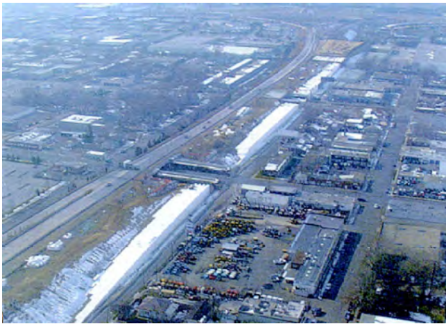
Figure 17.15 Aerial view of a portion of the I-15 project under construction, Salt Lake City, UT. Courtesy of AFM Corporation.
