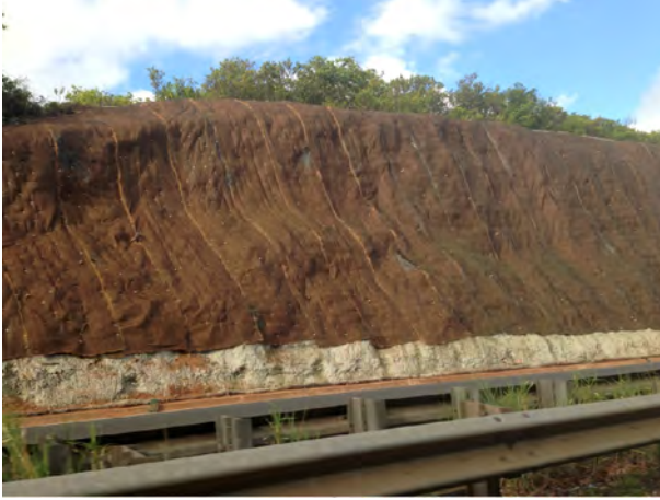
Figure 14.27 Pinned reinforcement mat for stabilization (erosion control and sloughing) of shallow, surface soils of steep roadcut, Kailua, HI.
