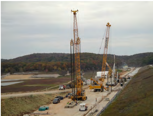
Figure 7.2 Installation of a 60 m (200 ft) deep slurry cutoff wall at Clearwater Dam, Piedmont, MO. Courtesy of Layne Christensen.
