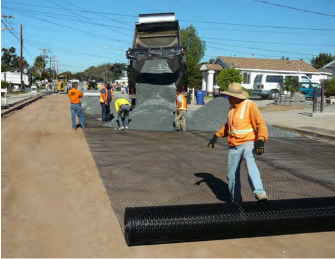
Figure 14.25 Triaxial geogrid beneath base coarse for a paved roadway. Courtesy of Tensar International Corp.
