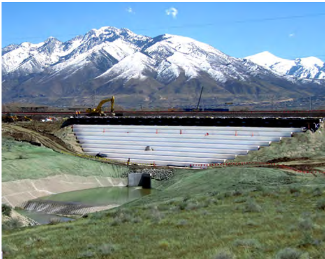
Figure 17.5 Commuter rail embankment over a box culvert, Draper, UT. Courtesy of ACH Foam Technologies.
