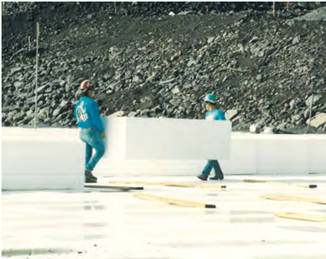
Figure 17.1 Geofoam blocks. Courtesy of Geolabs Hawaii.
