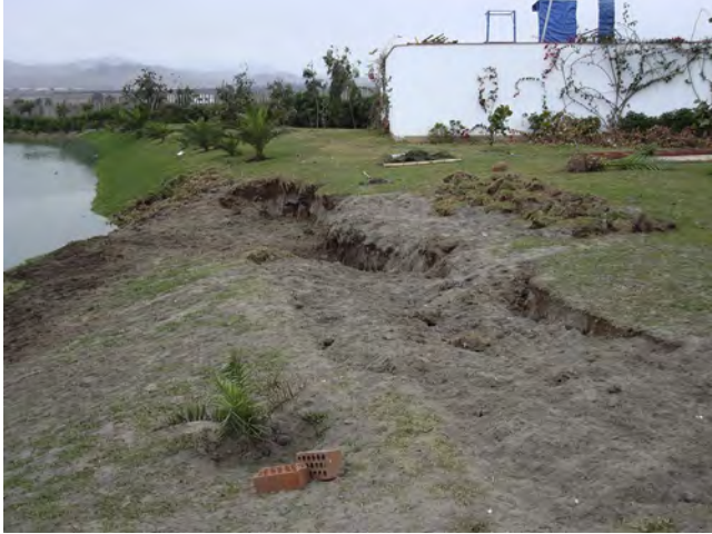
Figure 3.11 Liquefaction-induced lateral spreading. Courtesy of GEER.
