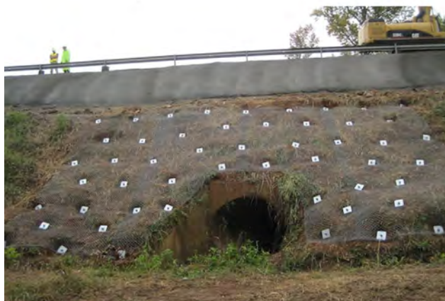
Figure 16.31 Slope stabilization incorporating anchored and tensioned netting to provide confinement. Top: After Koerner, 2005; Bottom: Courtesy of GeoStabilization International.
