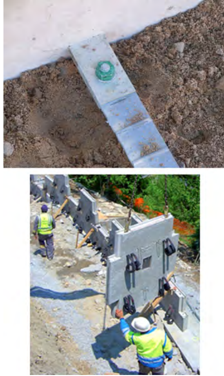
Figure 14.11 Typical wall connections for precast facing panels. Courtesy of The Reinforced Earth Company.
