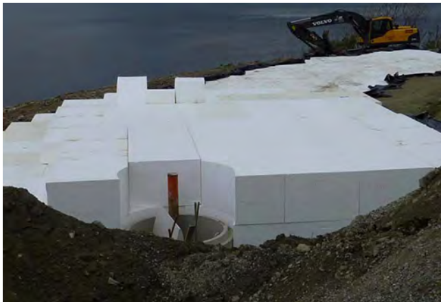
Figure 17.9 Cut and shaped geofoam fit around a drainage conduit. Courtesy of Atlas EPS.
