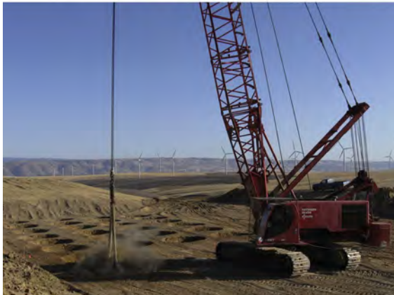
Figure 6.13 Photos of DDC field applications. Courtesy of Hayward Baker (top) and Densification, Inc. (bottom).
