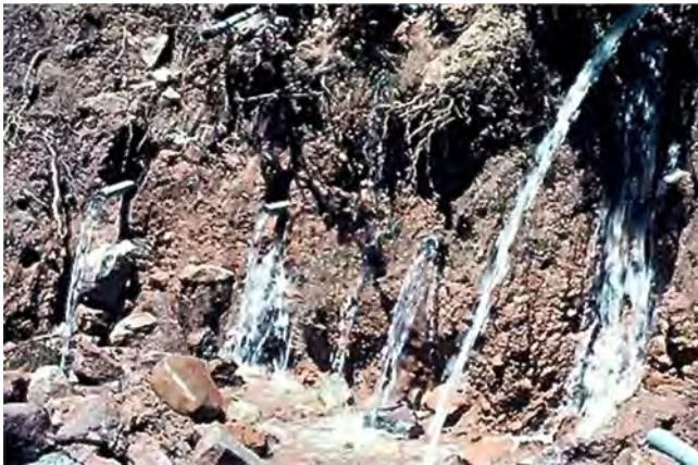
Figure 7.14 Drainage of a slope with closely spaced launched horizontal drains. Courtesy of GeoStabilization International.
