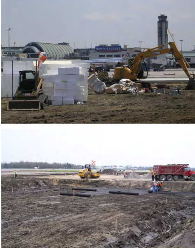
Figure 17.18 Geofill application for expanded taxiway at Louis Armstrong International Airport, New Orleans, LA. Courtesy of AFM Corporation.
