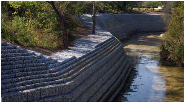
Figure 16.8 Gabion (buttress) retaining wall construction schematic. Courtesy of Hayward Baker.
