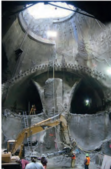
Figure 7.6 Application of deep wells to dewater for a deep shaft and tunnel excavation at Beacon Hill, WA. Courtesy of Moretrench.
