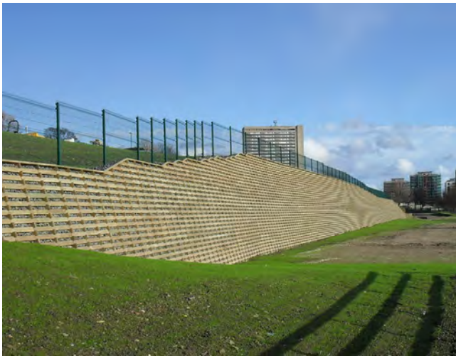
Figure 16.7 High concrete crib wall. Courtesy of Maccaferri, Inc.
