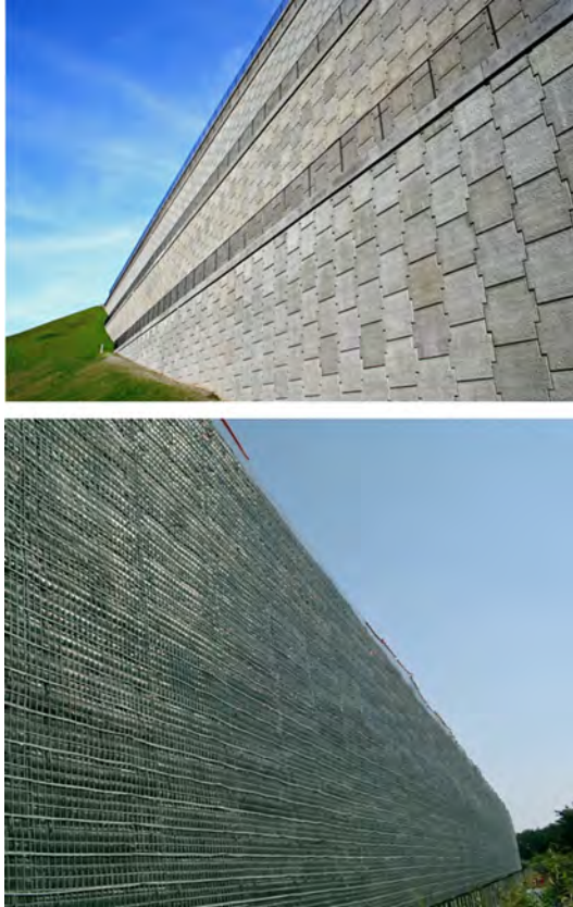
Figure 14.10 Example of some wall facings: top—precast panels, bottom—wire-wrapped. Courtesy of The Reinforced Earth Company.
