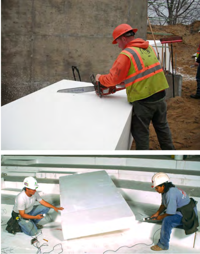
Figure 17.8 Cutting and shaping Geofoam blocks with a chainsaw (above) and hot wire saw (below). Courtesy of Atlas EPS.
