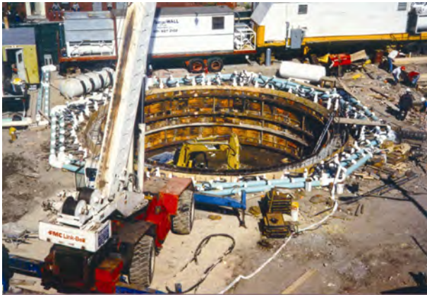
Figure 13.3 Freezing around the periphery of a deep-shaft construction. Courtesy of Moretrench.
