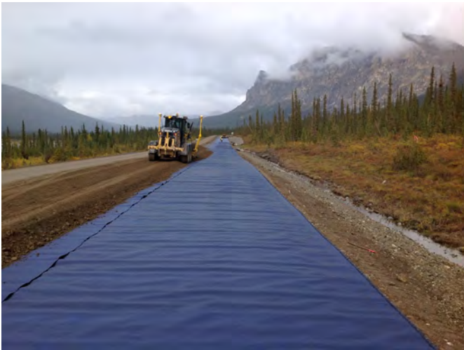
Figure 14.23 Geotextile for unpaved roadway reinforcement. Courtesy of Tencate-Mirafi.
