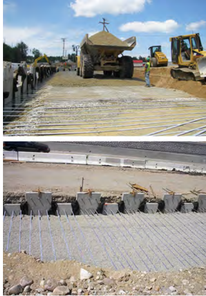
Figure 14.2 Construction of a metallic strip reinforced wall. Courtesy of The Reinforced Earth Company.
