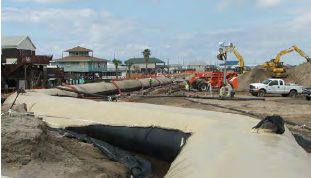
Figure 16.27 Construction of sand filled geotubes for a hurricane protection (storm surge) barrier. Courtesy of Infrastructure Alternatives, Inc.
