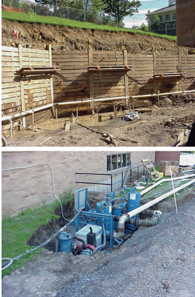
Figure 7.5 Wellpoint application and pump for a building excavation, Colgate University, NY. Courtesy of Moretrench.
