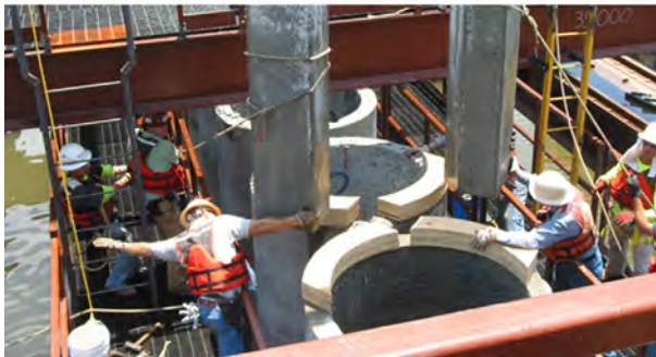
Figure 12.18 Jet grouted assisted pile installation and closure IHNC MRGO. Courtesy Layne Christensen.
