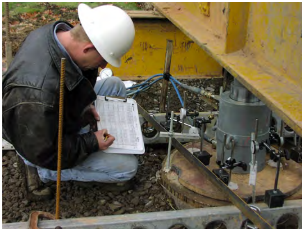
Figure 6.22 Field load test of a Geopier ® system. Copyright by Geopier Foundation Company, Inc. Reprinted with permission.
