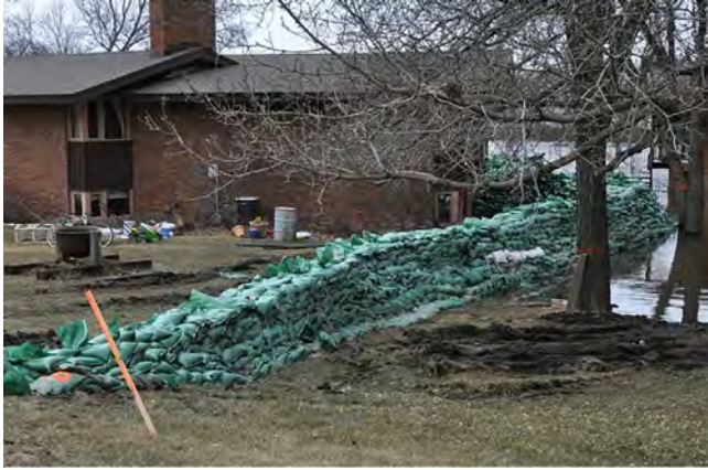
Figure 16.1 Use of sandbags as a temporary “earthen” flood control levee. Courtesy of FEMA.
