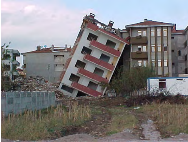
Figure 3.9 Liquefaction-induced bearing capacity failure. Courtesy of GEER.
