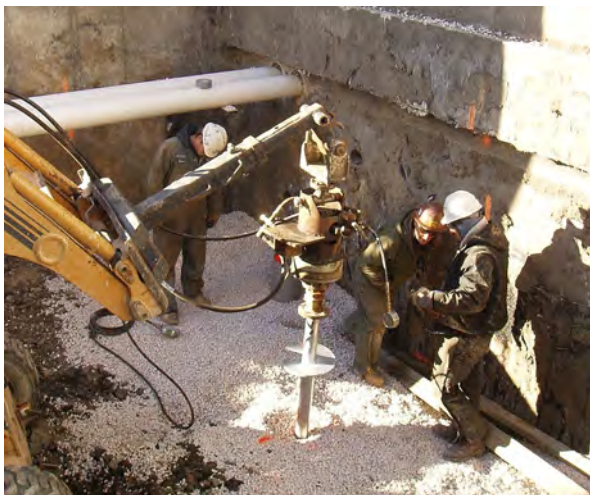
Figure 15.15 Installation of a helical pier. Courtesy of Hayward Baker.
