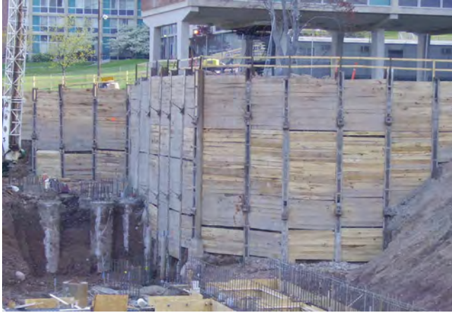
Figure 15.1 Ground anchor supported soldier beam and lagging excavation wall. Courtesy of Hayward Baker.
