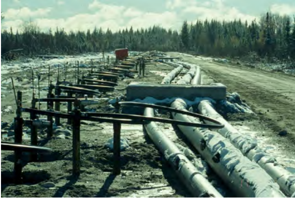
Figure 13.14 Ground freezing for (2.5 mi) perimeter barrier around the Aquarius Gold Mine, Timmins, Ontario, Canada. Courtesy of Layne Christensen.
