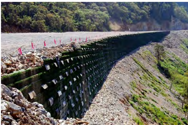
Figure 14.12 Geosynthetic wrapped-face wall. Courtesy of Tencate-Mirafi.
