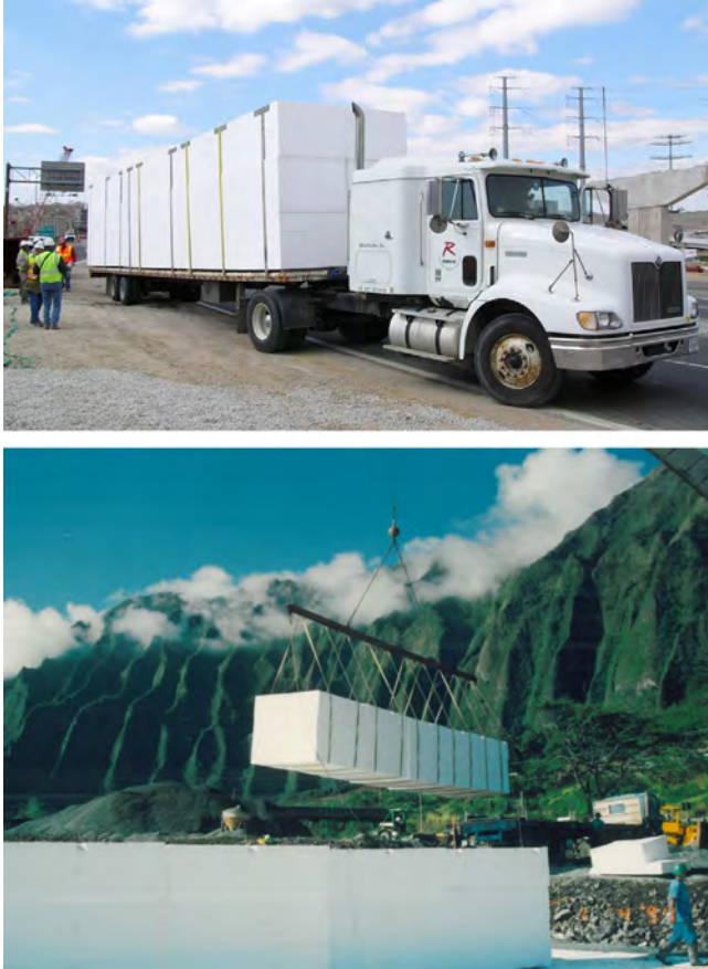
Figure 17.7 Bulk Geofoam site delivery. Top courtesy of FHWA; bottom Courtesy of Geolabs Hawaii.
