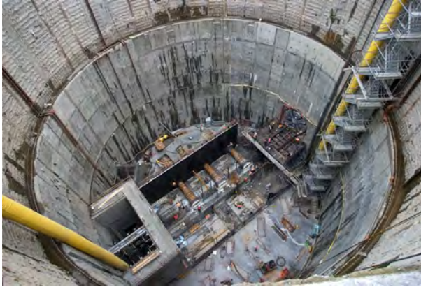
Figure 12.13 Deep shaft with jet grouted cut-off plug for sewer pump station in Portland, OR. Courtesy Layne Christensen.
