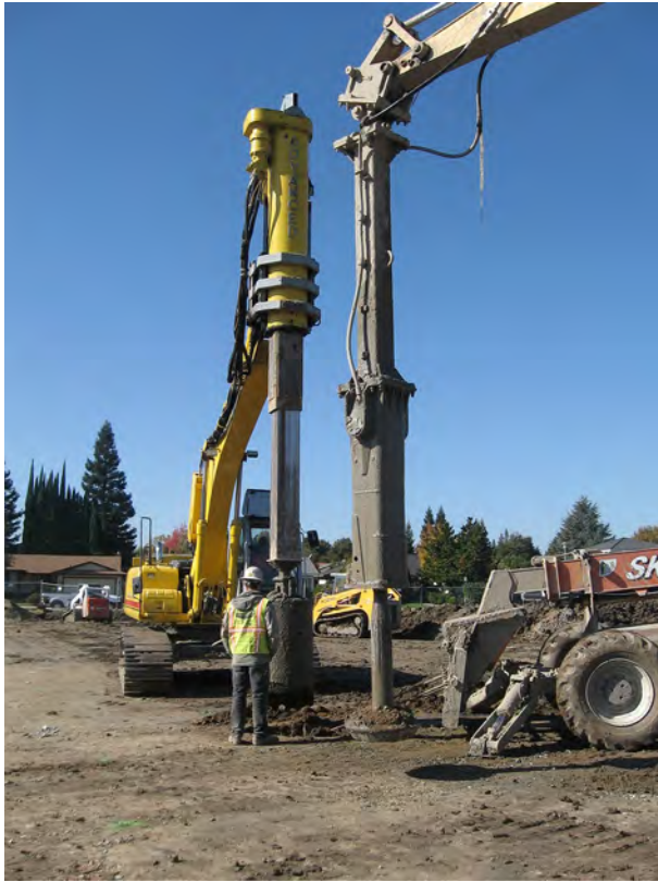
Figure 6.9 Equipment used for installation of a Rammed Aggregate Pier® system. Courtesy of Geopier Foundation Company, Inc.
