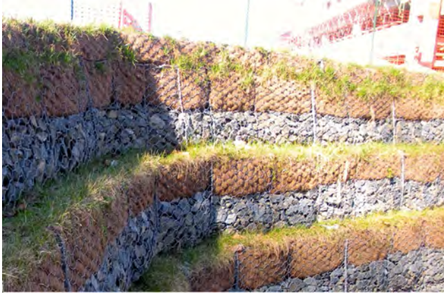
Figure 16.10 “Green” gabion wall. Courtesy of Maccaferri, Inc.
