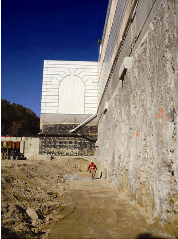
Figure 12.9 Continuous jet grout wall underpinning an existing building. Courtesy of Hayward Baker.
