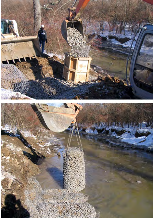
Figure 16.13 “Sack gabion” being filled and placed in water. Courtesy of Maccaferri, Inc.
