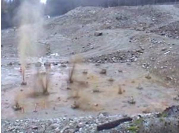
Figure 6.1 Example of field blasting showing expulsion of excess pore water. Courtesy of Explosive Compaction, Inc.
