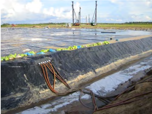
Figure 9.11 Field application of vac consol. Courtesy of Menard USA.
