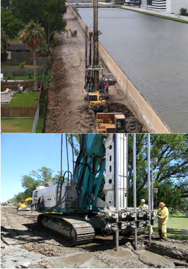
Figure 12.10 Triple axis jet grouting for rehabilitation of 17th Street levee in New Orleans, LA. Courtesy of Layne Christensen.
