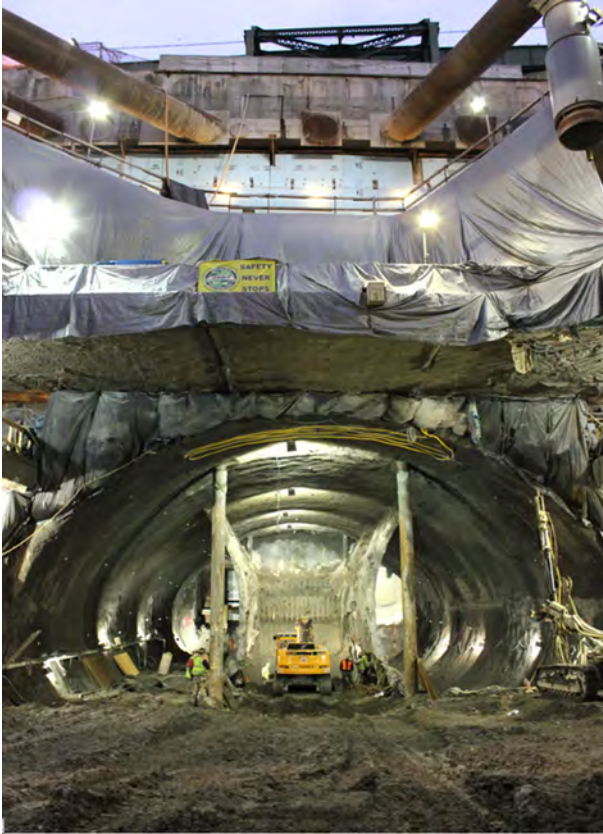
Figure 13.12 View of the complex conditions for tunneling through frozen ground beneath urban infrastructure. Courtesy of Moretrench.
