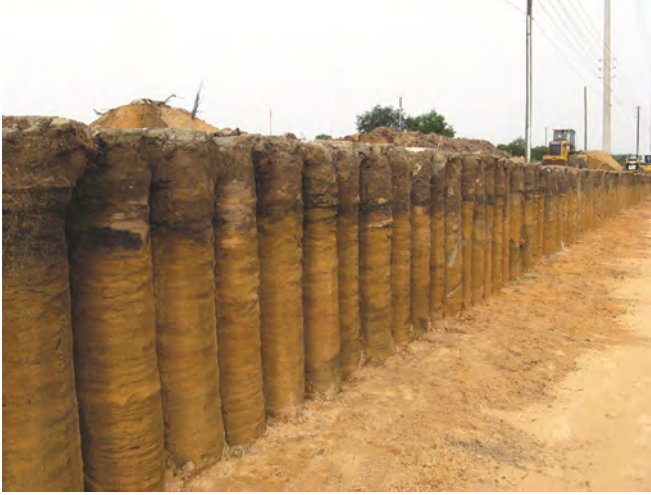
Figure 11.13 Excavated soil-lime column wall. Courtesy of Hayward-Baker.
