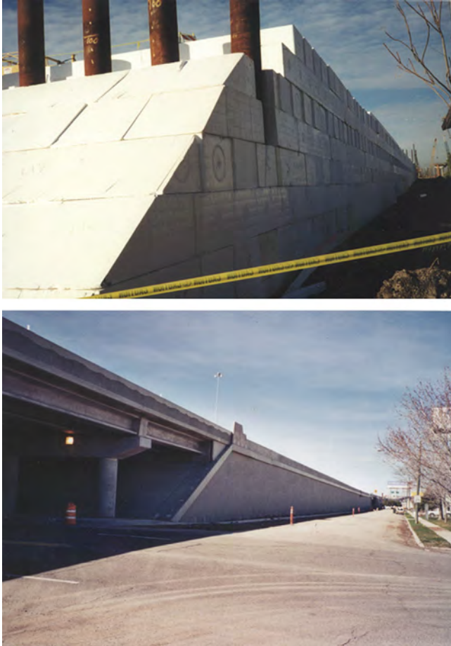
Figure 17.16 During and after construction of bridge abutment for I-15 project, Salt Lake City, UT. Courtesy of AFM Corporation.
