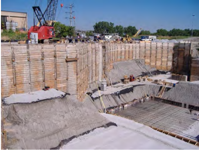
Figure 16.4 Photo of a soldier piles and lagging excavation support. Courtesy of Hayward Baker.
