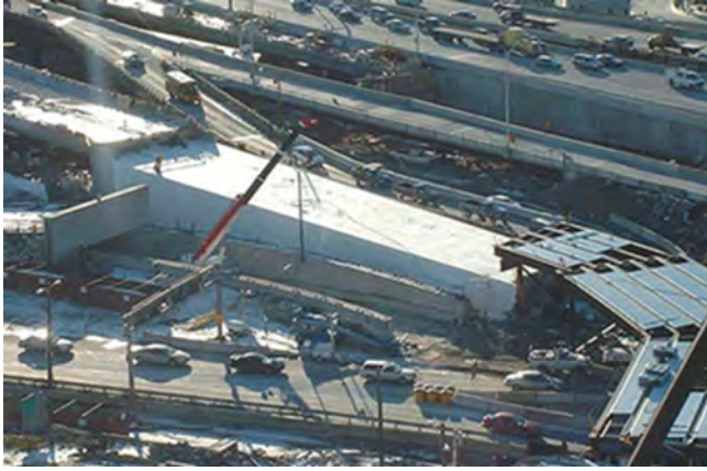
Figure 17.14 Use of Geofoam for a highway ramp as part of reconstruction of Boston's Central Artery ("Big Dig") project. Courtesy of FHWA.
