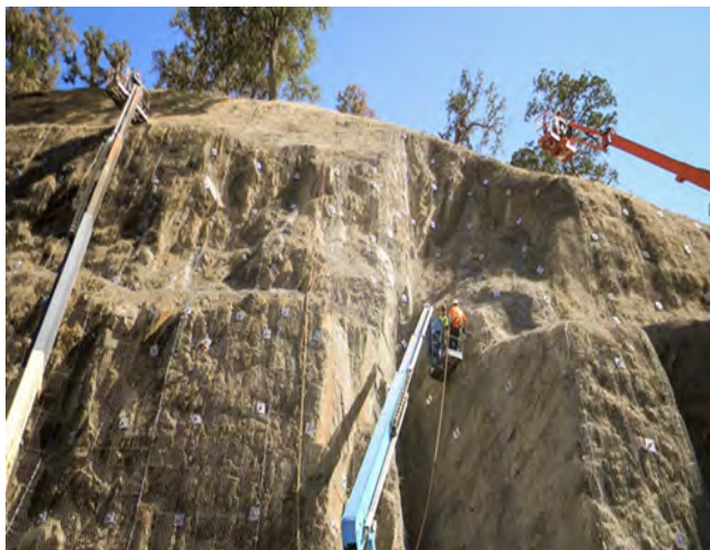
Figure 16.30 Confinement of weathered rock face with steel mesh and soil nails. Courtesy of GeoStabilization International.
