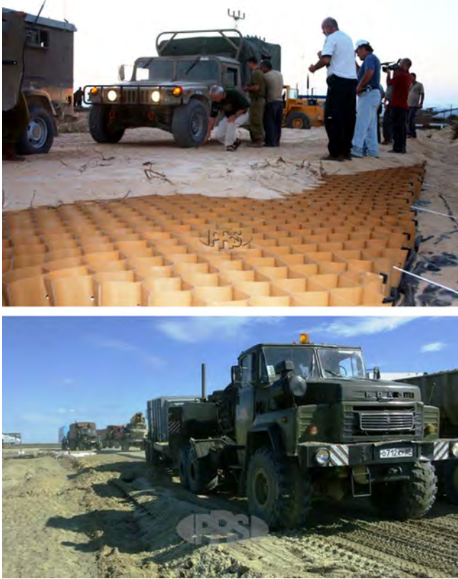
Figure 16.22 Geocells used in rapid road construction for military mobilization in desert environments. Courtesy of PRS Mediterranean Ltd.
