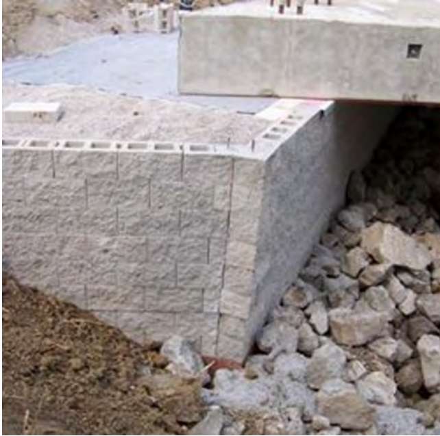
Figure 16.24 Geosynthetically reinforced wall with light concrete facing blocks. Courtesy of Federal Highway Administration.
