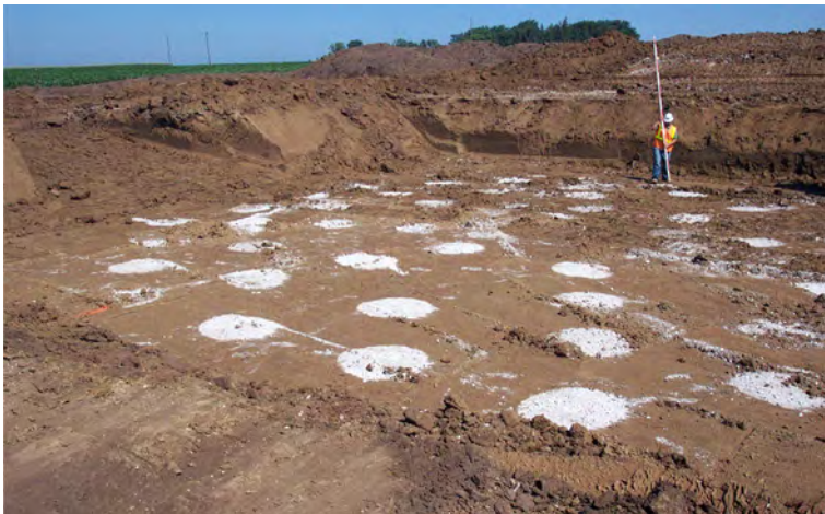
Figure 6.11 Geopier ® reinforced site. Copyright by Geopier Foundation Company, Inc. Reprinted with permission
