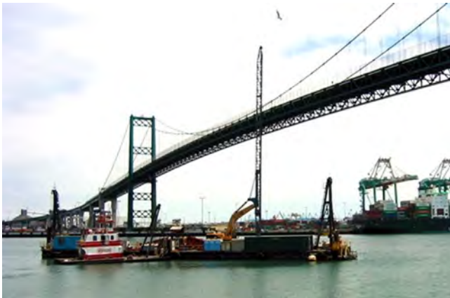
Figure 9.8 PVD install underwater (Port of Los Angeles). Courtesy of Hayward Baker/HB Wick Drains.
