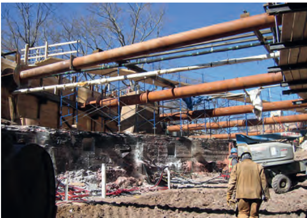
Figure 7.7 Application of ejector wells to dewater for a deep excavation at the South Ferry Terminal, NYC. Courtesy of Moretrench.
