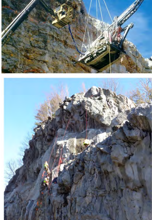
Figure 15.8 Rockfall mitigation with nails/rock bolts. Top: Courtesy of Layne Christensen; Bottom: Courtesy of GeoStabilization International.
