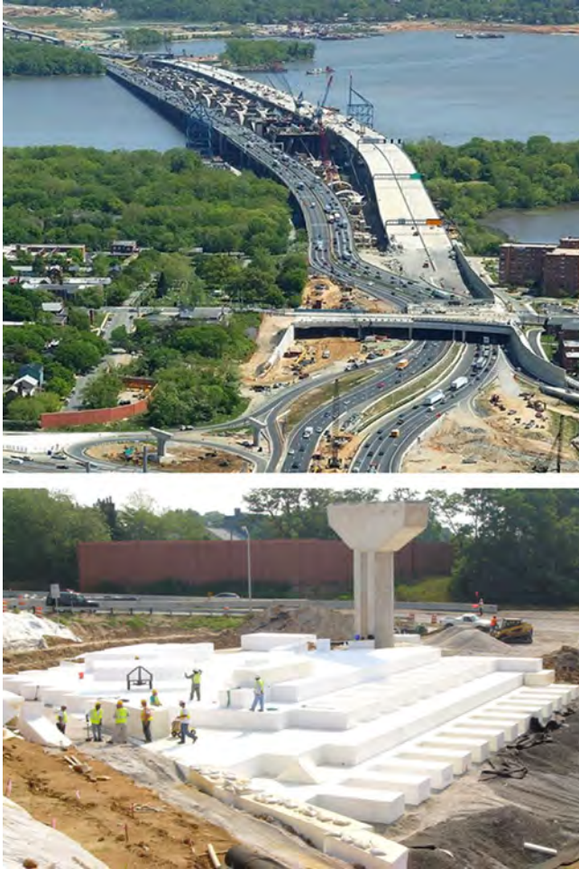
Figure 17.13 Construction of the new Woodrow Wilson Bridge, approach, and interchanges. Courtesy of FHWA.
