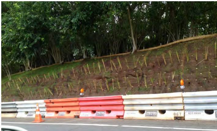
Figure 14.30 Reinforced steep slope surface with vegetation “plugs.”
