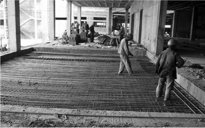
Figure 1.10 GFRP reinforced-concrete slab (Oran, Algeria).
