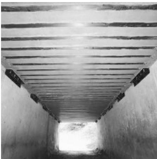
Figure 11.27 Completed bonding operation of underpass, Great Missenden.
