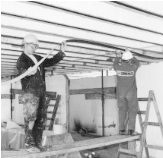
Figure 11.3 Positioning an 11.0m laminate to underside of rib.
