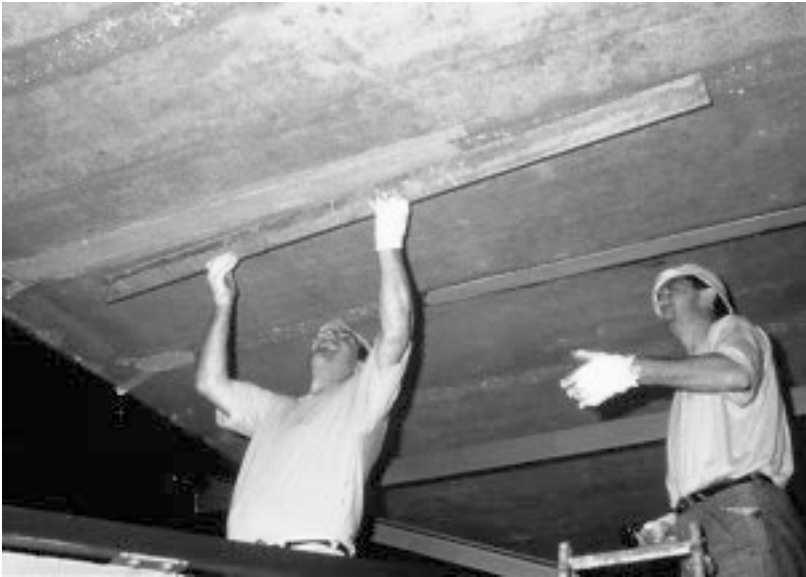
Figure 11.13 Checking the evenness of the reprofiled surface.
