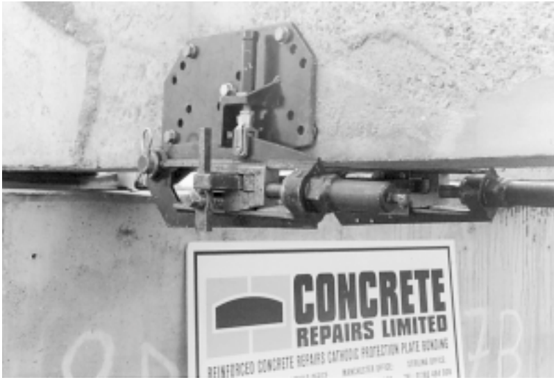
Figure 10.7 Prestressing machine bolted in place to a reinforced concrete beam.
