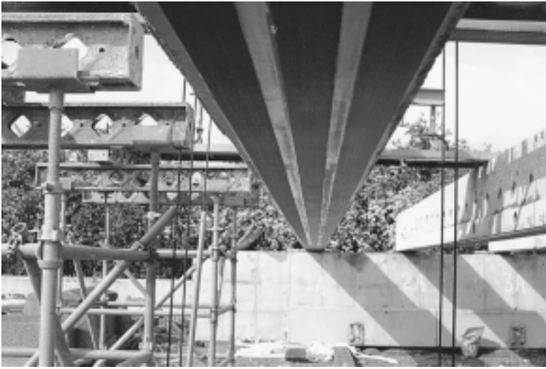
Figure 10.12 Overall view of completed installation of plates to a reinforced concrete bridge beam.
