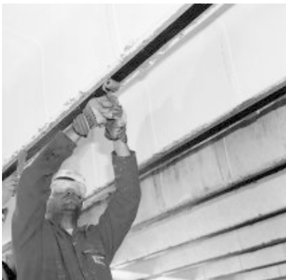
Figure 11.4 Bedding CarboDur laminate into adhesive with hand roller.
