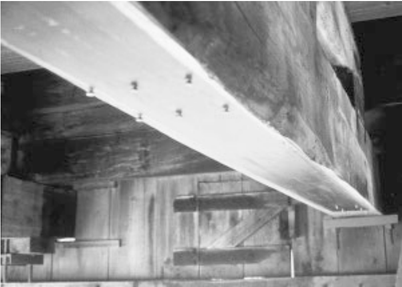
Figure 11.22 A close-up of the bonded plate to the underside of the beam.
