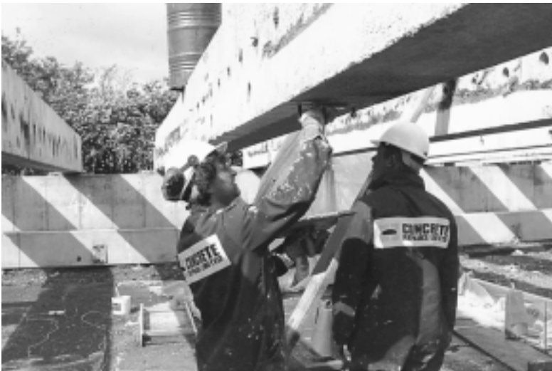
Figure 10.1 Applying epoxy adhesive to prepared concrete surface.
