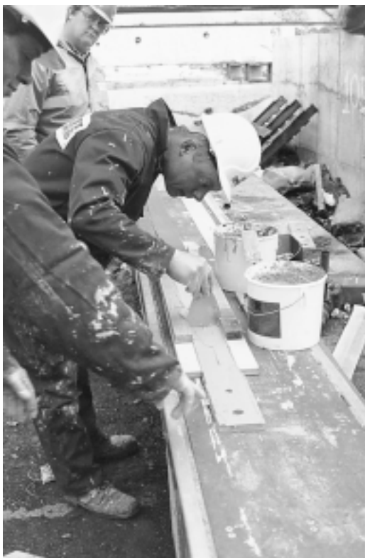
Figure 10.2 Setting dome-shaped spatula into adhesive reservoir prior to application of epoxy adhesive to plate.
