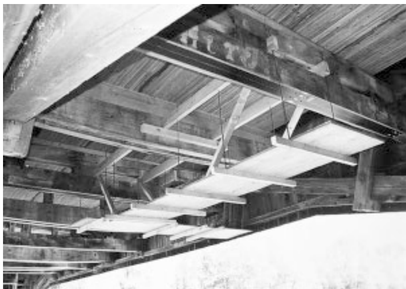
Figure 11.21 View of strengthened cross beams.
