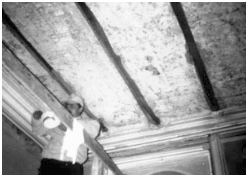
Figure 11.31 Application of CarboDur laminates.
