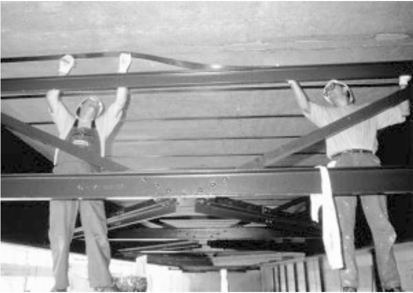
Figure 11.10 Installation of CarboDur laminate.
