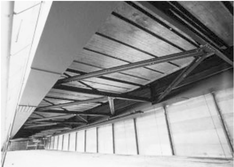
Figure 11.14 Completed strengthening work on Rhine bridge, Oberriet.
