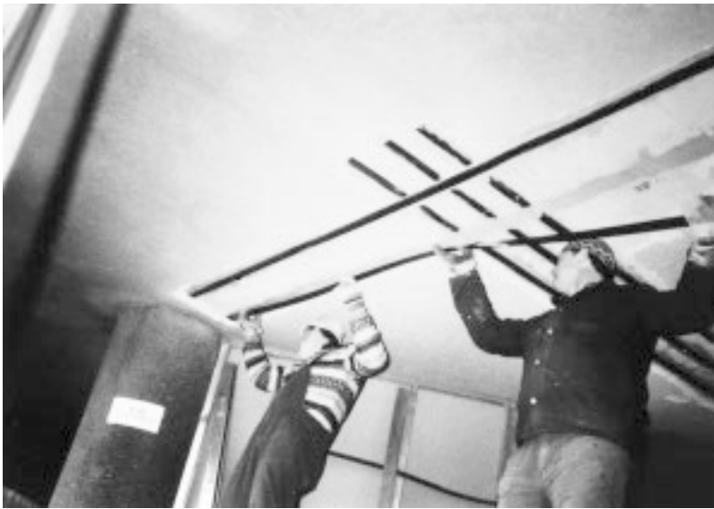
Figure 11.32 Application of CarboDur laminates.
