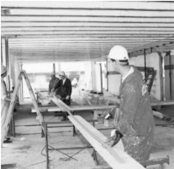
Figure 11.2 Application of adhesive to CarboDur laminate.
