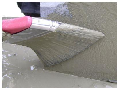
Polymer-modified Slurry Primer - PSP™
