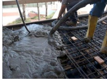
Mortar for Concrete Cathodic Protection- MCP™
