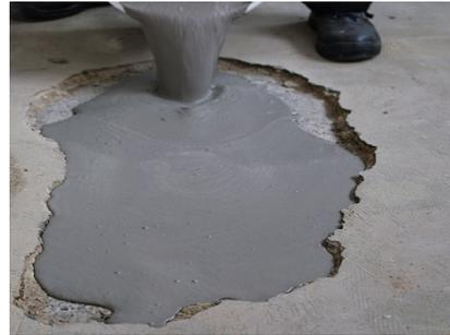
Pourable Polymer Modified Traffic Bearing Repair Mortar- TRM™200
