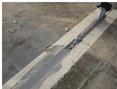
Polyurethane-based Swellable Waterstop- PSW™
